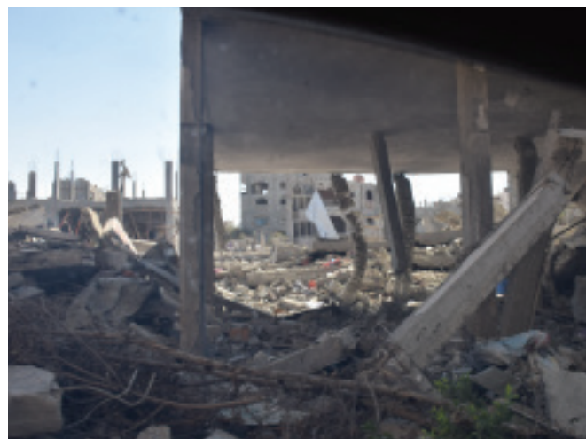
Another example of the difficulties of mapping damages from satellite imagery. The building in front can look intact from above.
