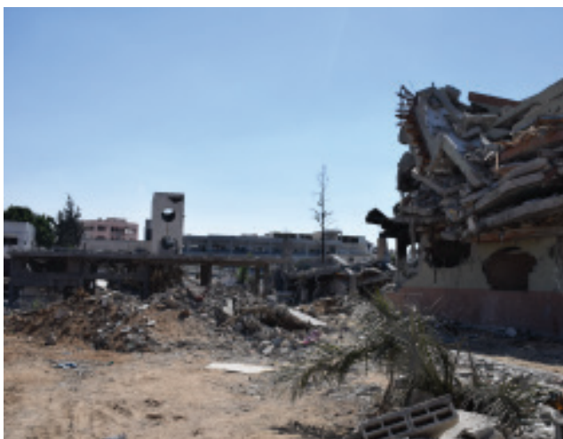
On the right: a building classified as severely damaged but not destroyed by UNOSAT. A partially destroyed gov. school in the back.
