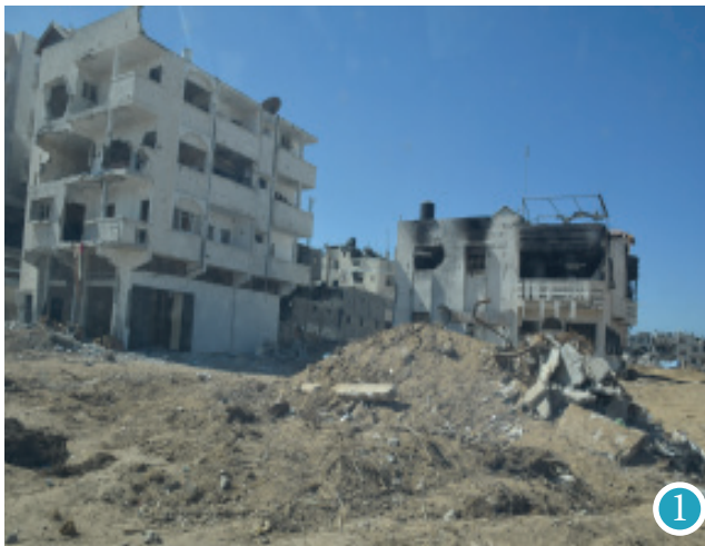
The building to the left is mapped as severely damaged, while the 2 floor building to the right is moderately damaged.
